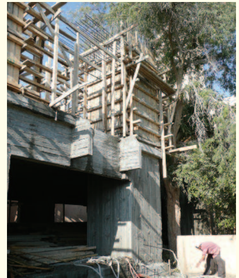
New Library under construction, May 2009
