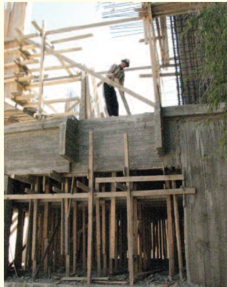
New Library under construction, April 2009
