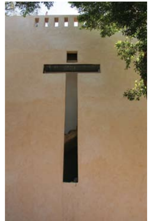
Lighting the stairs!
